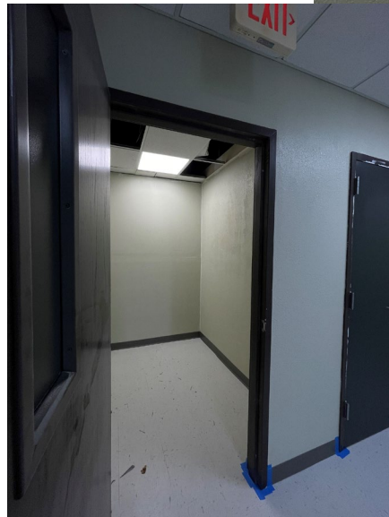
The odd, side hallway entrance to the Senior Room has been enclosed, creating much needed janitorial storage
